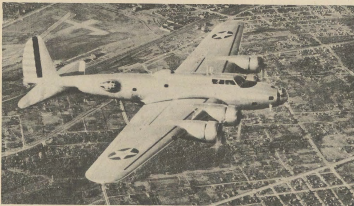
THE B-17A WENT HIGHER: Equipped with turbos, it topped all previous service ceilings, gave maximum performance above 30,000 ft. To range, speed, bomb load, firepower, the B-17 added another advantage: altitude operation.
